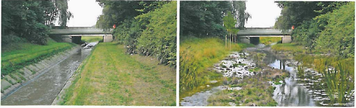
Figure 31: Emscher re-conversion at the Berne (left side: technical state, right side: one year after restoration) (Source: Johann & Frings, 2016).
