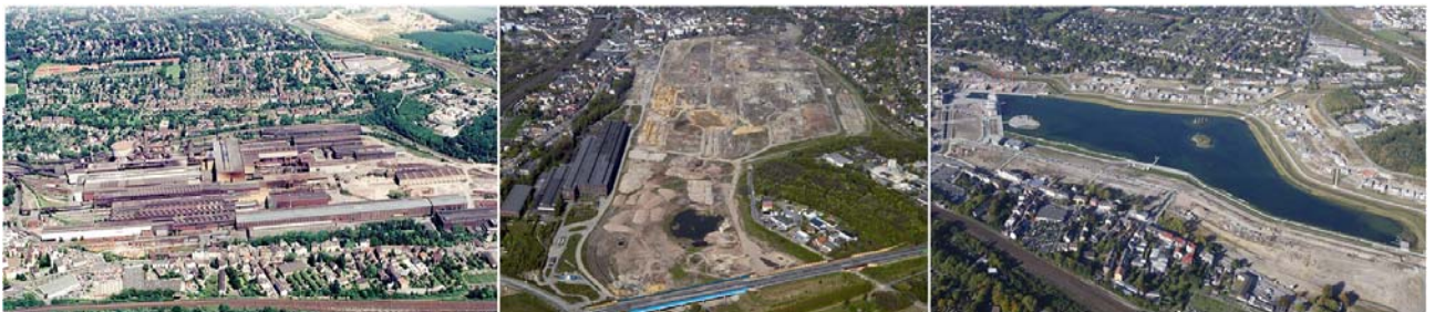
Figure 41: Creation of Lake Phoenix (left: steel processing plant at the area of Phoenix East, center: Phoenix East area after plant dismantling, right: completed creation of Lake Phoenix) (Source: EGLV, Hans Blossey)
