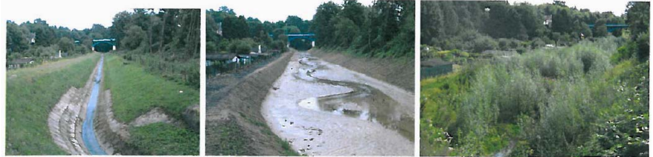
Figure 12: Emscher re-conversion at the Borbecker Mühlenbach. left side: technical state, middle: directly after restoration, right side: two years after restoration (Source: Johann, Frings 2016).
